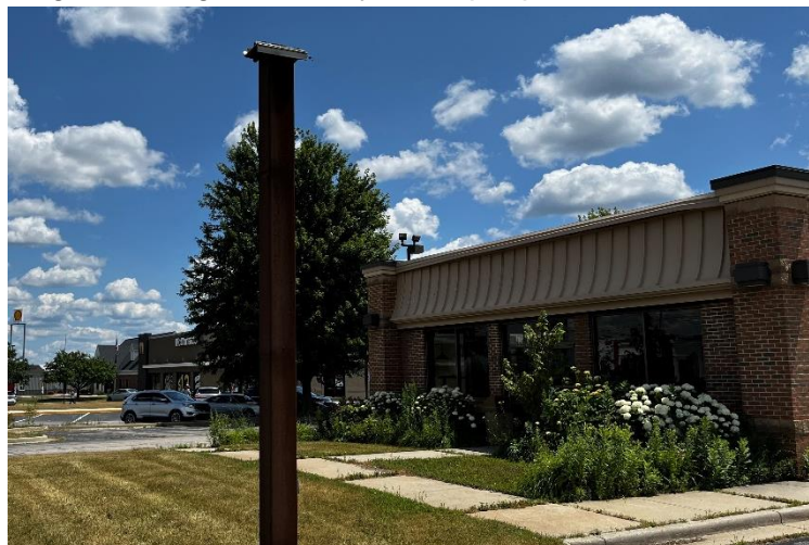
Vacant Commercial Building on Business 127
